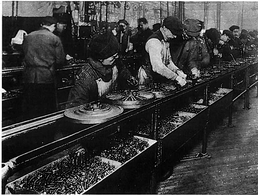
The Highland Park Ford Plant in Michigan, where the automated assembly line was first introduced in 1913.
